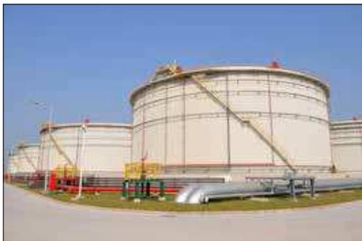
CP in the form of a sacrificial anode or an impressed current is often used to protect the bottoms of aboveground storage tanks from corroding and eventually leaking. However, variations in the floor of the tanks, such as irregularities caused by uneven bending of the tank bottom as the tank is filled or emptied, may limit the effectiveness of the CP by leaving certain areas out of reach of the CP current delivered through the tank base.
